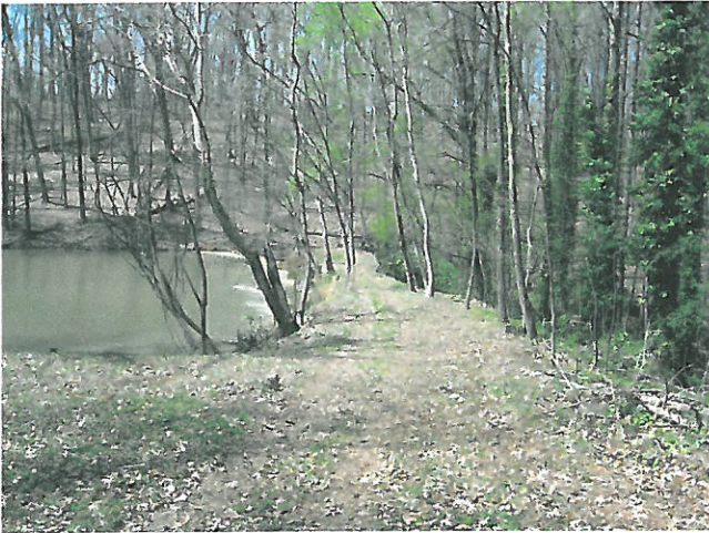
1. Crest of dam.
