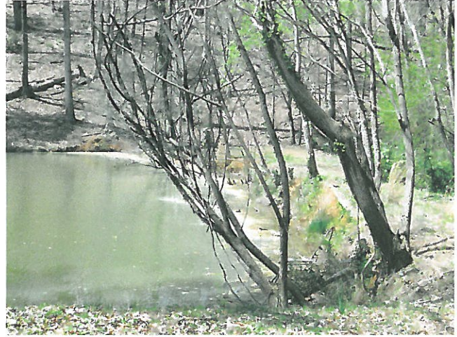
2. Front slope of dam.
