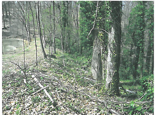
6. Back slope of dam.
